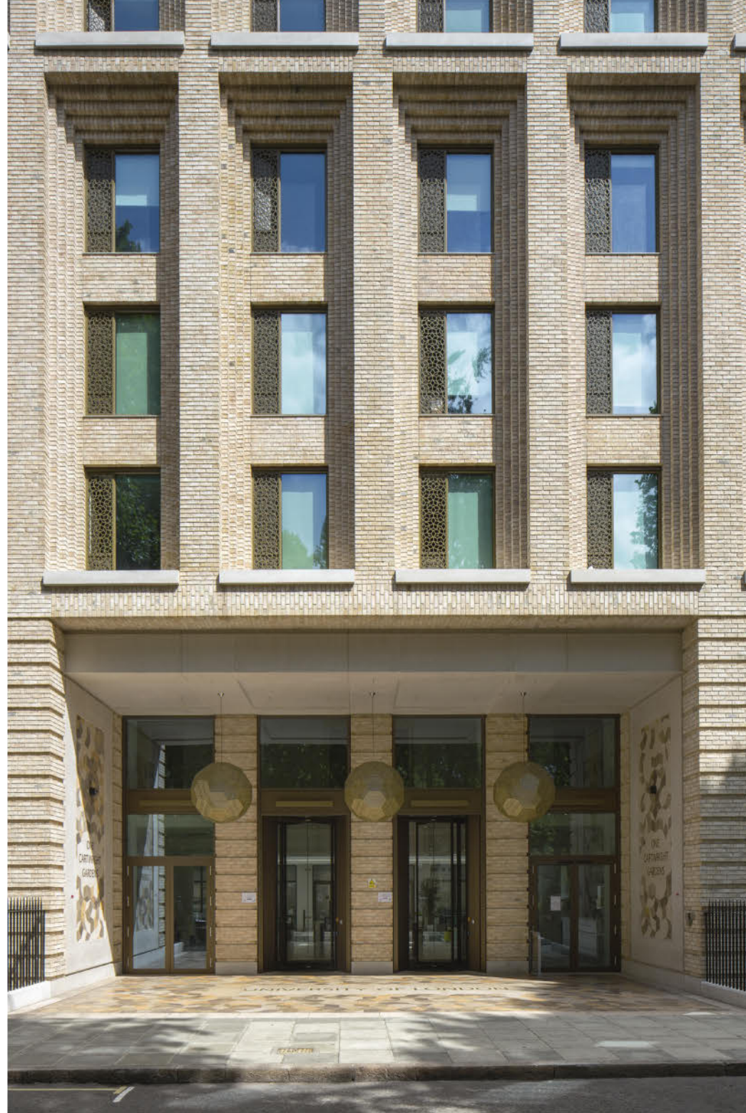
The entrance facing Cartwright Gardens is drawn back from the façade, where four high doorways lead into the building.
