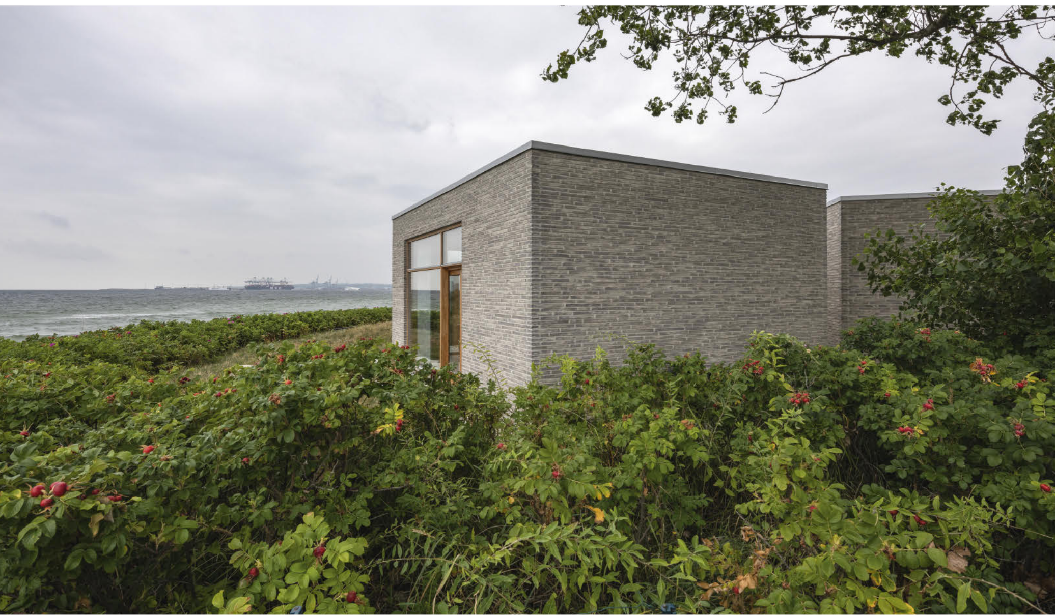
The prominent position called for a muted approach to both design and idiom. The architect and builder were inspired by the colours of the surrounding landscape, and opted for natural materials that age beautifully.
