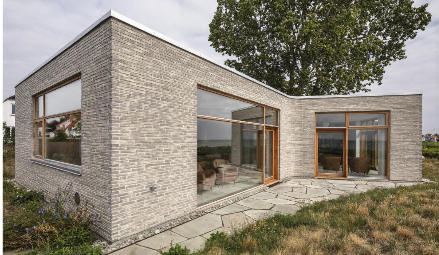
Large windows open up the house to the south and west. The doors and windows are made of oak, the terraces of slate. The quality of the bricks means that the façade can go all the way down below ground level.
