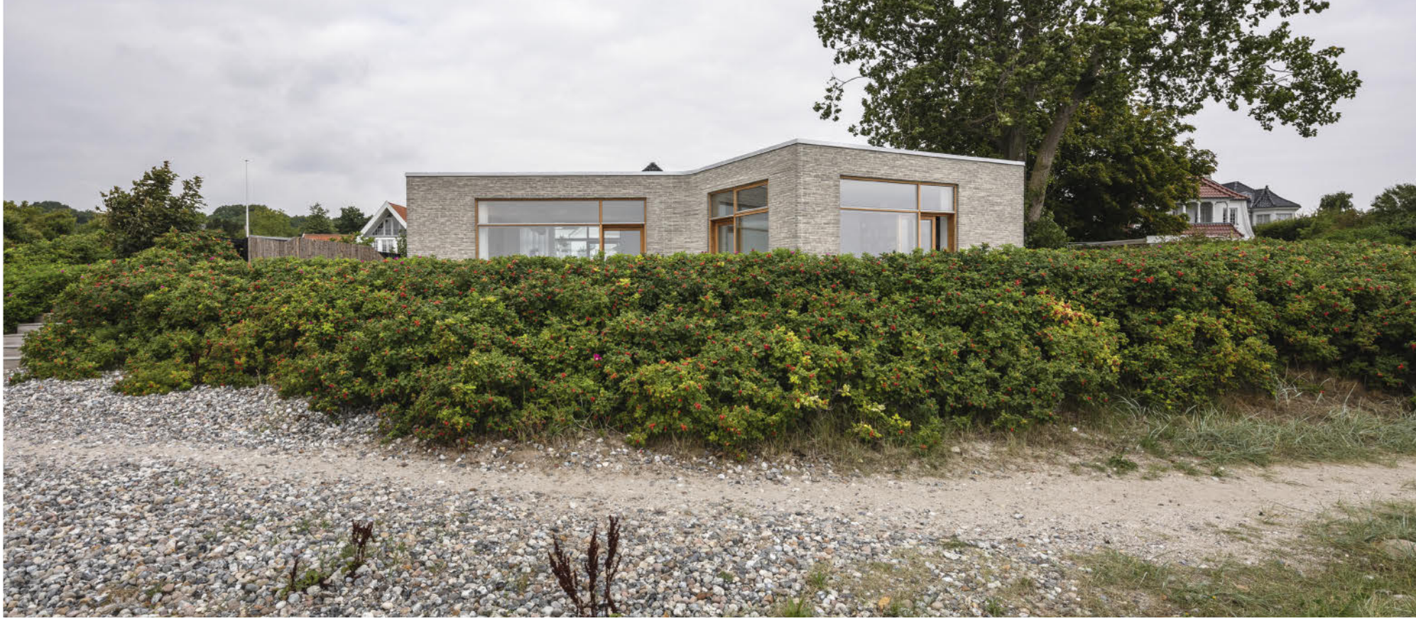
Villa Platan stands a few metres from the water's edge, just north of Aarhus. Early in the process, the architect and clients took brick samples to the beach to find the grey-white play of colour that most closely resembled the shades of the sand and pebbles.
