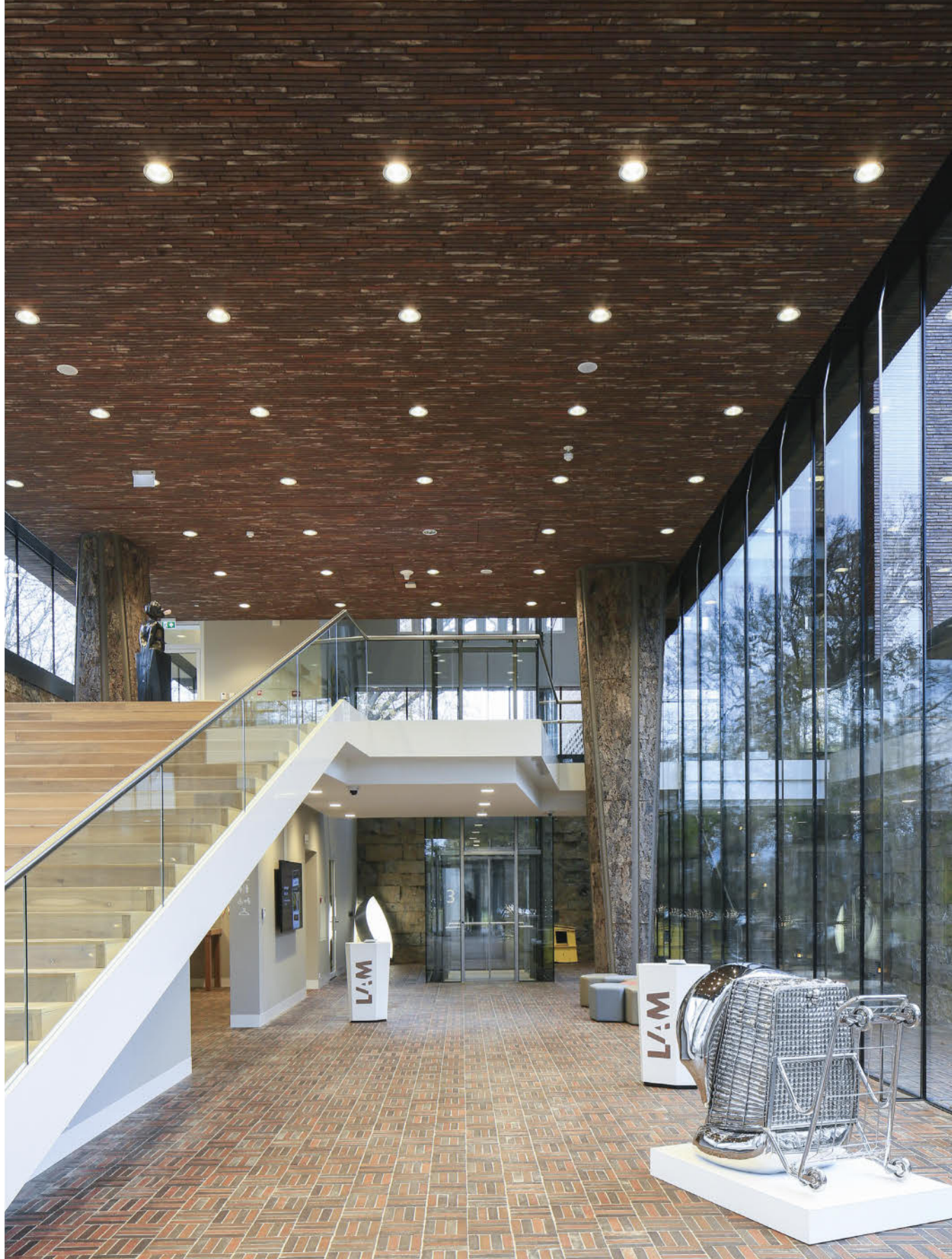
The entrance to the museum is below the cantilevered wing, where a wide staircase leads up to the exhibition hall. The ceiling in the big glass entrance hall is clad in the same brick as the façades.
