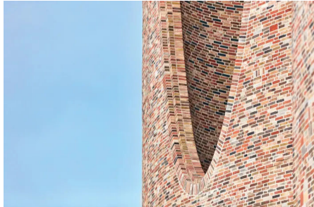
15 shades of “D” bricks at the Fjordenhus, Jutland
