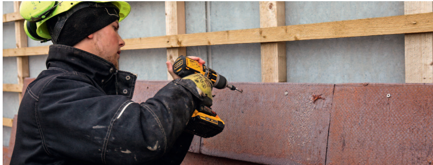
Fitting Petersen Cover is approximately 20% faster than traditional bricklaying with brick and mortar.
