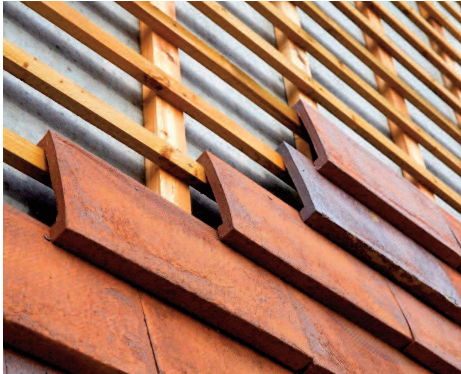
Fitting Petersen Cover is approximately 20% faster than traditional bricklaying with brick and mortar.
